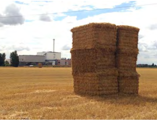
Glennmont's 38 MW straw-fired biomass plant in the UK
