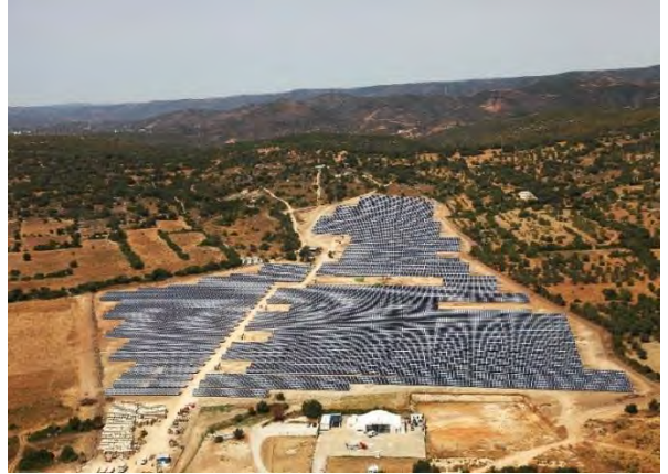
Part of Glennmont's 48 MW solar park portfolio in Portugal
